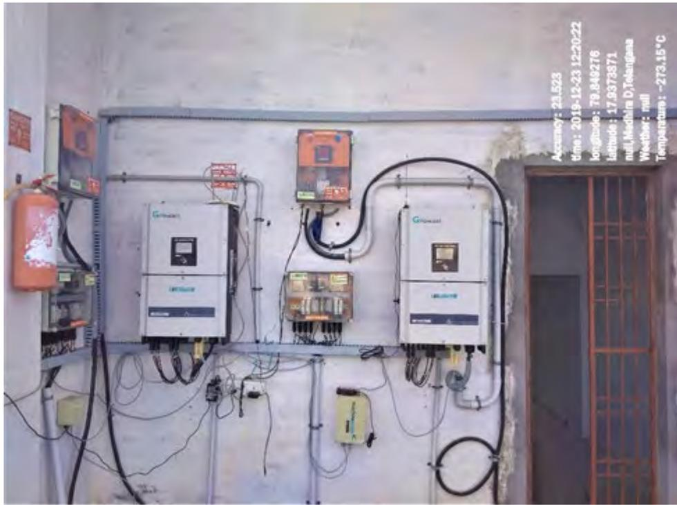
Image: Roof top solar PV plant-Inverter- BITS Block
